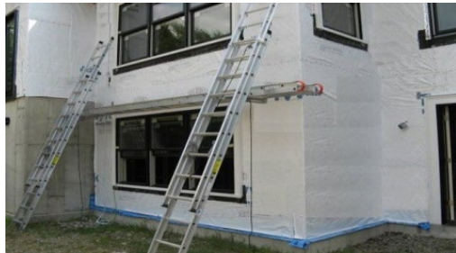
Ladder Jack Scaffold
